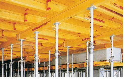
Installation of KAUFMANN HT 20 plus formwork beams
